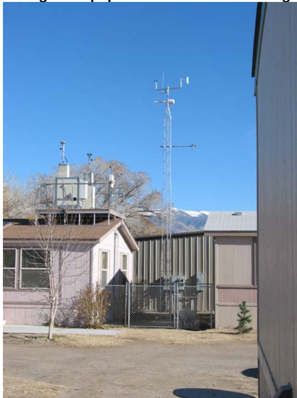
Photographs 1. Meteorological Equipment and Air Monitoring Platform and Location
